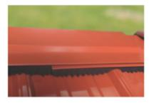
2. When installing, be sure to have the screws positioned at edge of the roof cap so the fasteners pass through the Flovent<sup>™</sup>. When overlapping ridge cap, cut the Flovent<sup>™</sup> back 12" to 18".
