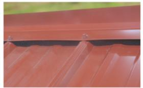
3. Fasten the ridge cap with the Flovent™ staying in place by the adhesive. Install the ridge cap per the mfg instructions.
